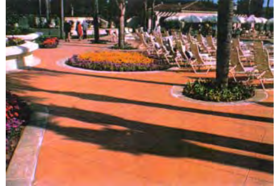
Example of colored concrete and granite edging that could be used at plazas and pedestrian passageways
