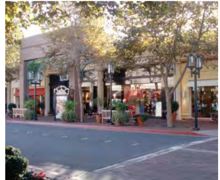
Example of decorative light fixture integrated into streetscape
