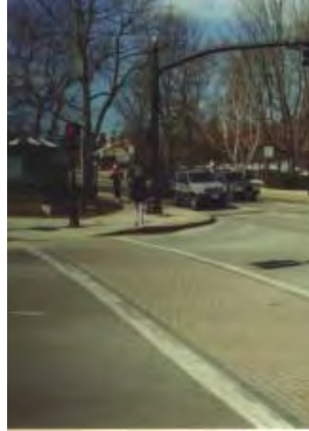
Example of precast brick pavers to delineate crosswalks
