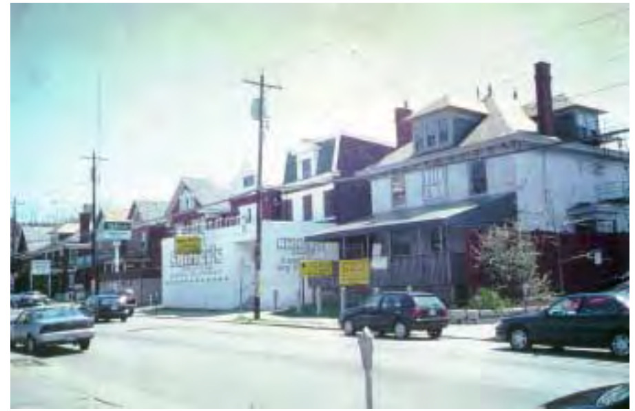
Example of poor store frontage along McMillan Street
