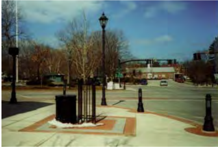
Example of paving accents (brick & granite) with granite curbing at typical sidewalks.
